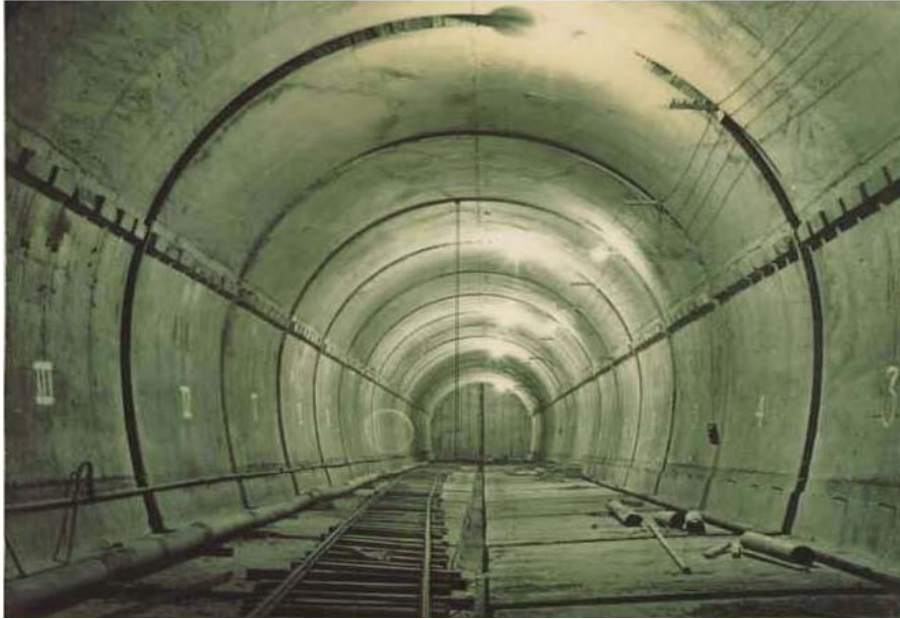
The interior of a tunnel during construction
