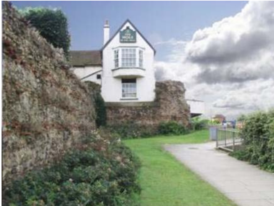
Hole In The Wall - Colchester
