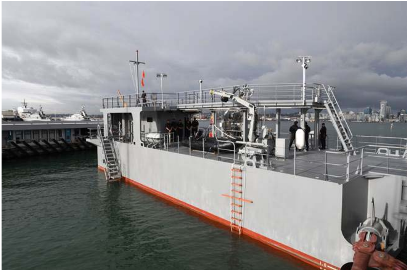
Seamanship Training Aid Facility - Waterside
