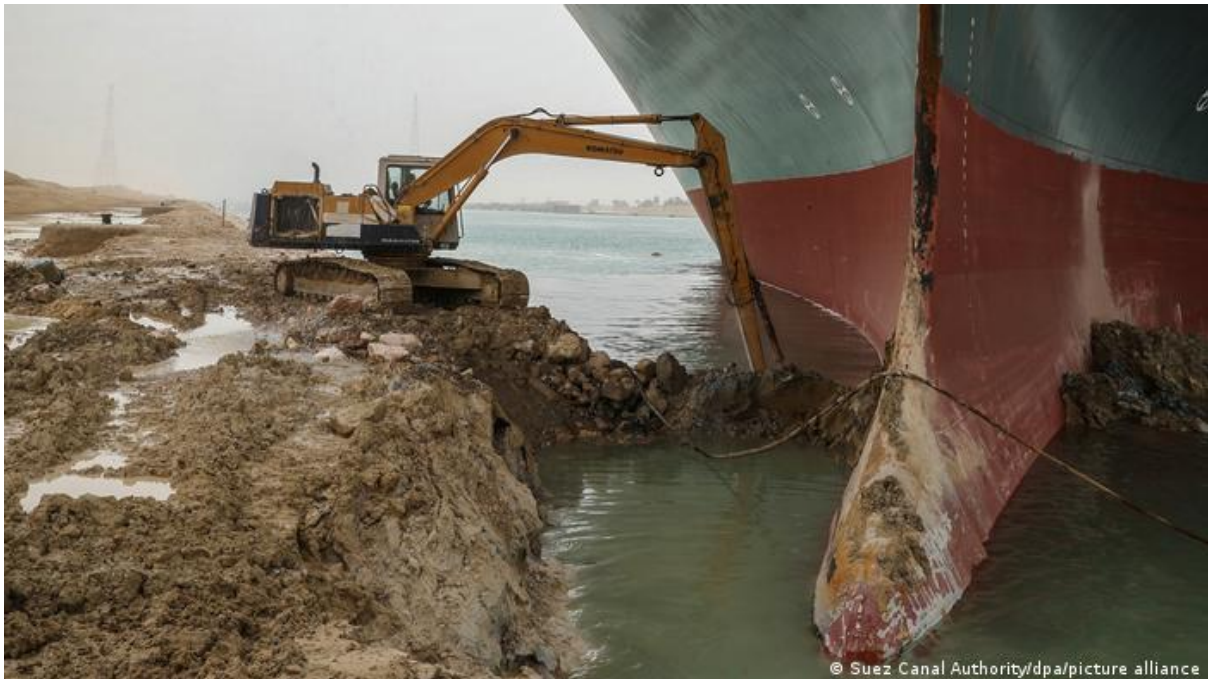
One man and his digger – frees a 200,000 tonne vessel
